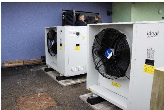
UK boiler manufacturer Ideal provided two Ecomod air source heatpumps for installation at Ysgol Tir Morfa as part of a field trial. The equipment uses air temperature and electricity to generate heat in place of a gas boiler. The efficiency of the system will help lower carbon emissions and costs compared to a traditional boiler. In addition to the
