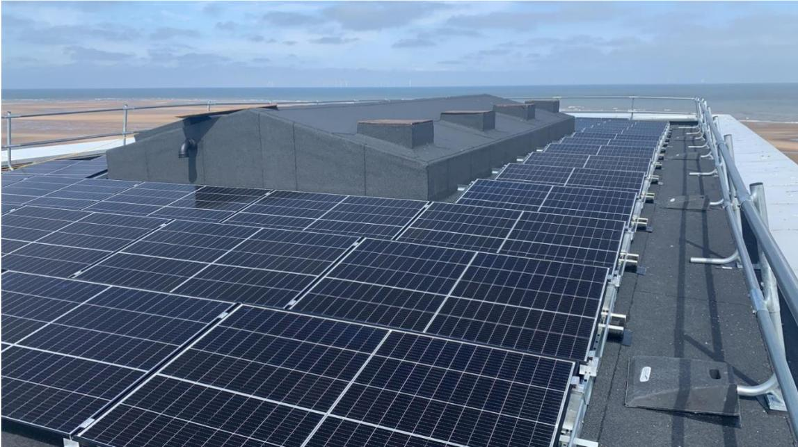
The project underway at **Betws Gwerfil Goch primary school** will show what can be achieved at sites not connected to the gas network. The oil boiler is being replaced with an Air Source Heat Pump. This is complemented by a solar PV array on roof and battery storage. The project will decrease the carbon emissions at the site by 7 tonnes per year.
